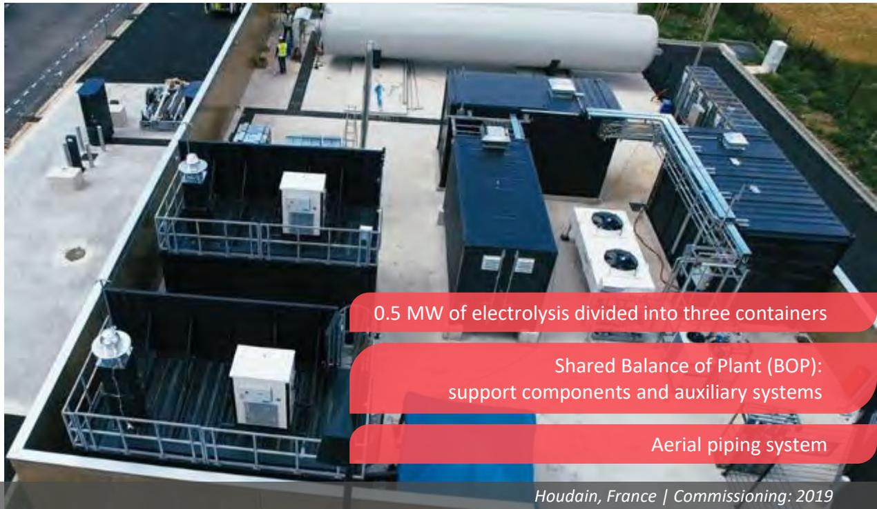
0.5 MW of electrolysis divided into three containers
