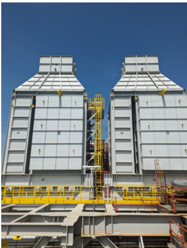
Figure 1 - Open Cycle Gas Turbine and LM2500+G4 GTG "Lean Package"
