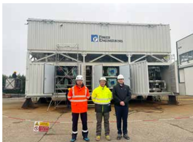
Figure 5: Electrolyzer in Fores construction site
