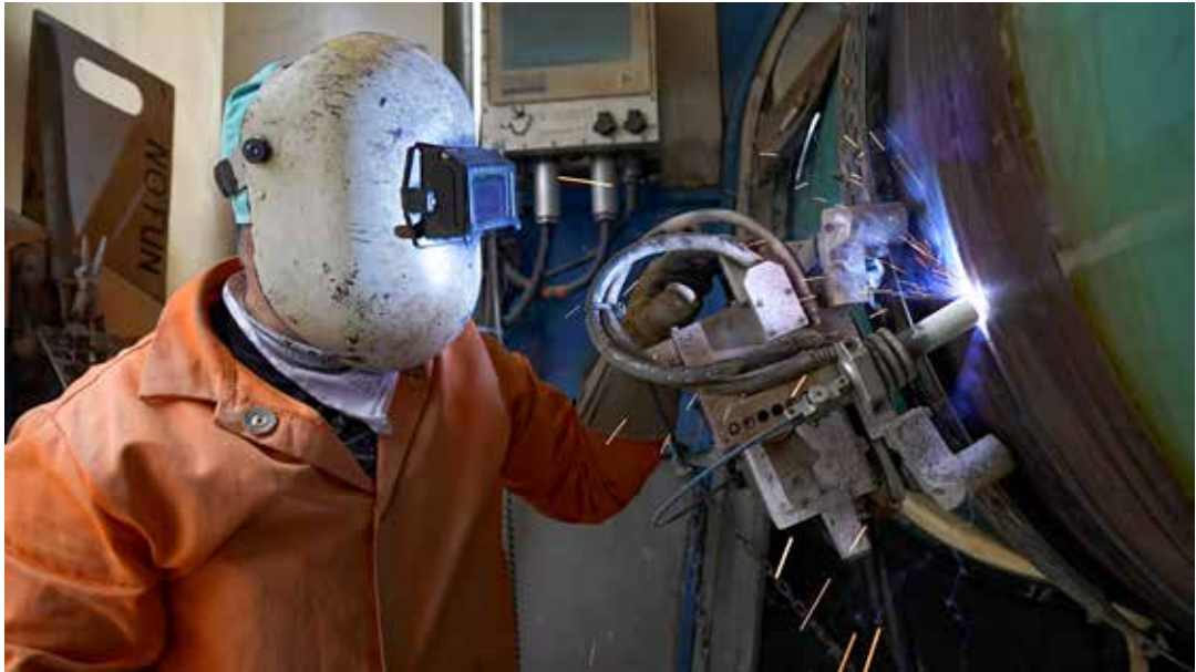
Bonatti's automated welding system in operation
