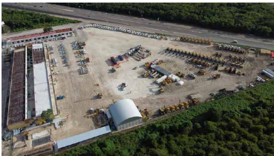
Cuxtal II Project, logistics base, Mexico
