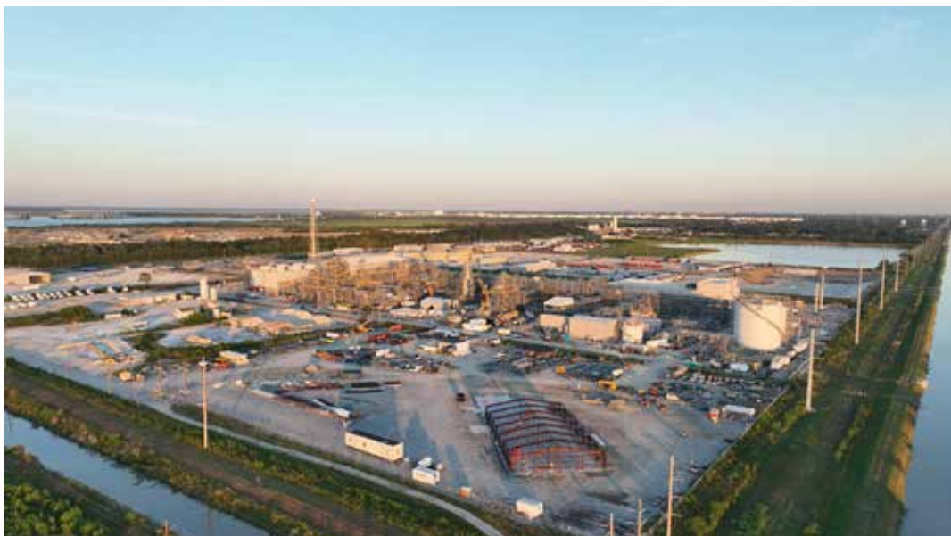
Blue Ammonia Synloop Plant Beaumont, USA
