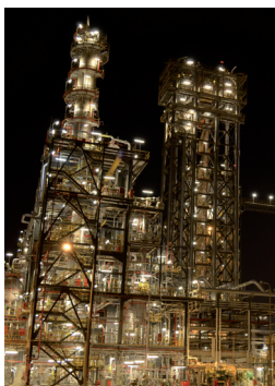
Stunning view of the Loop Reactor, core of the polymerization process facilities of the Polyethylene Plant - Borouge Polyolefins Complex, Ruwais, UAE
