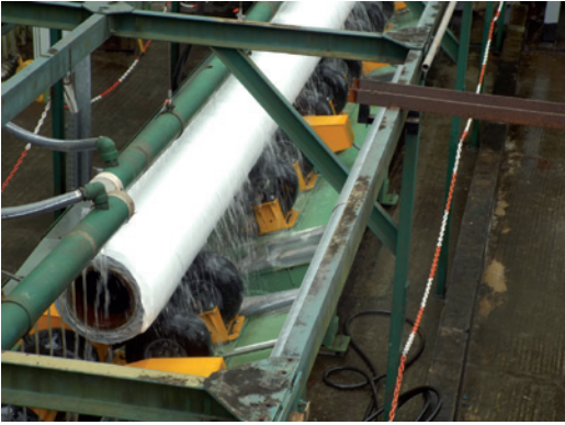
Fig. 8 – Coating at PCNL yard at Port Harcourt Onne area
