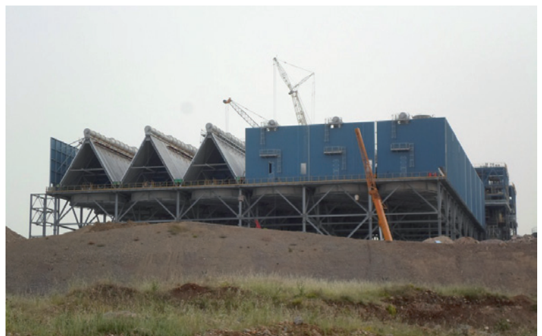
Fig. 7 - Construction phase of the ACC
