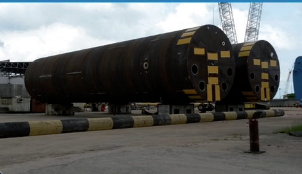
Fig. 10 – FPSO anchoring piles at Saipem's yard in Port Harcourt
