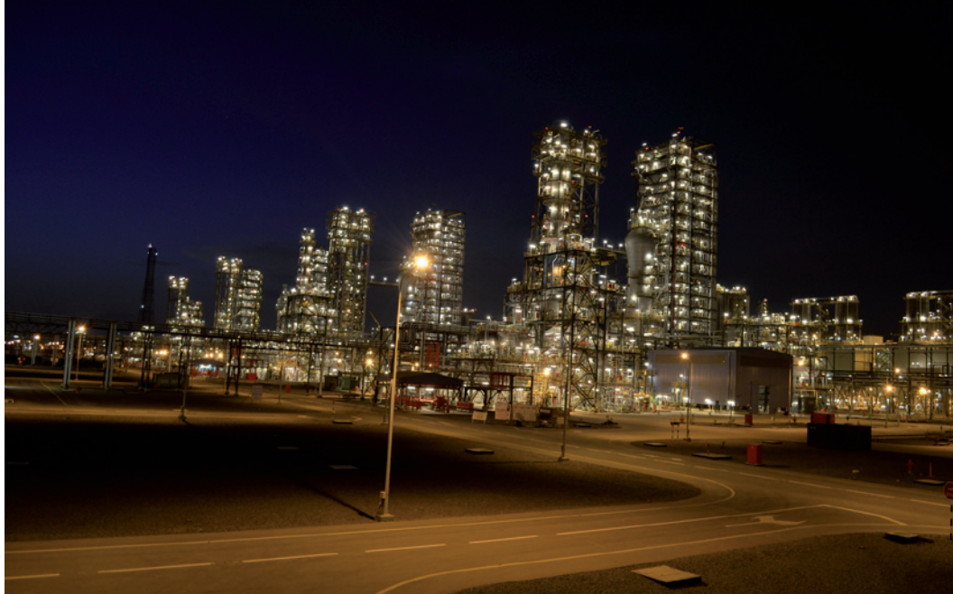
Fig. 8 - Night overview on the polyethylene and polypropylene polymerization areas
