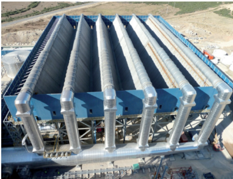
Fig. 4 - Spig environmentally friendly air cooled condenser
