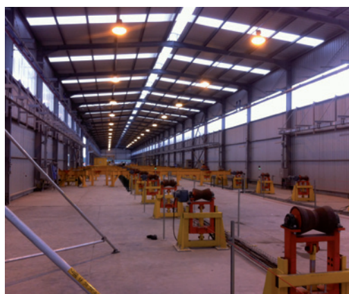
Fig. 6 – The Quad and Double Jointing plant
