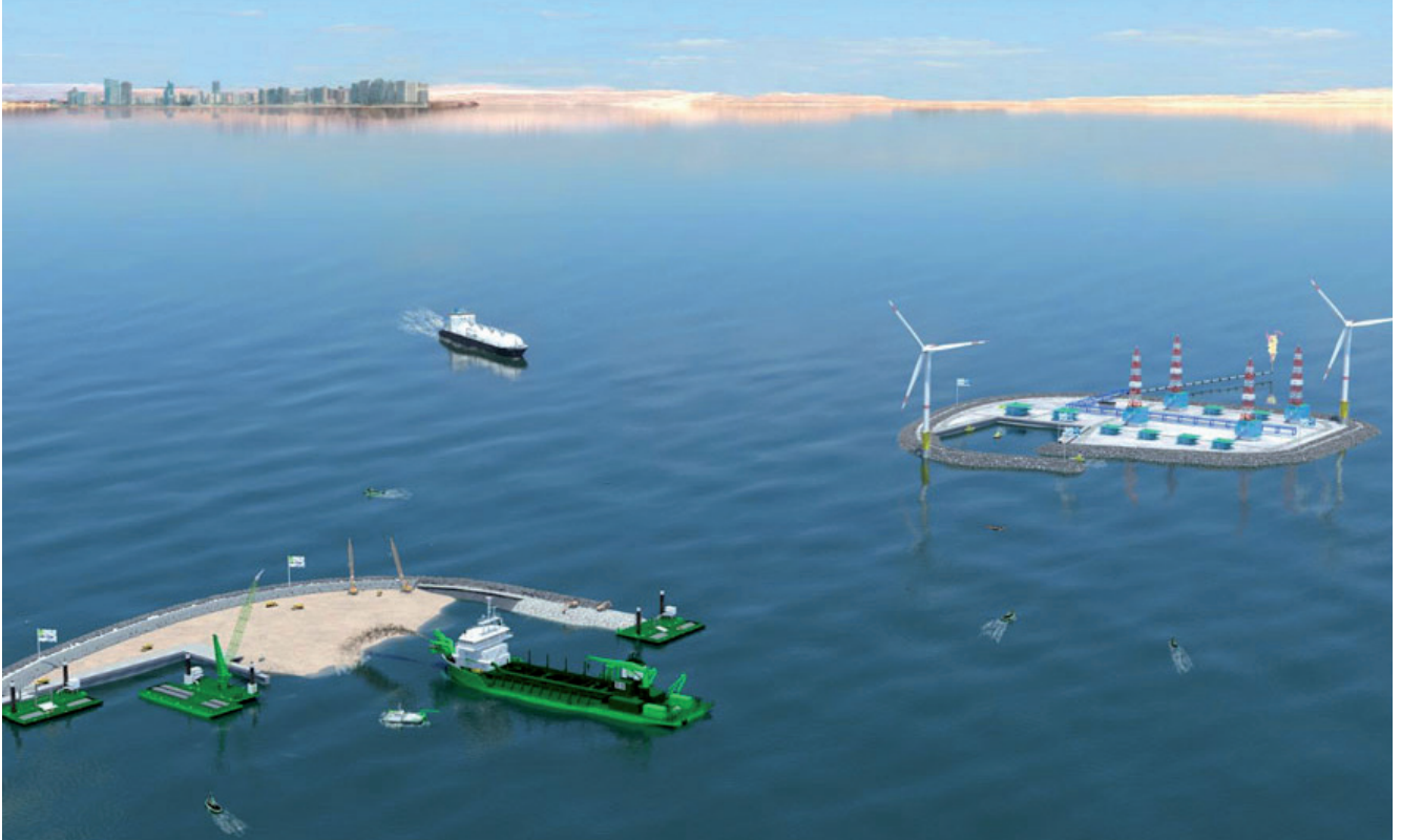
Fig. 3 - Sarb 1 & Sarb2 artificial islands
