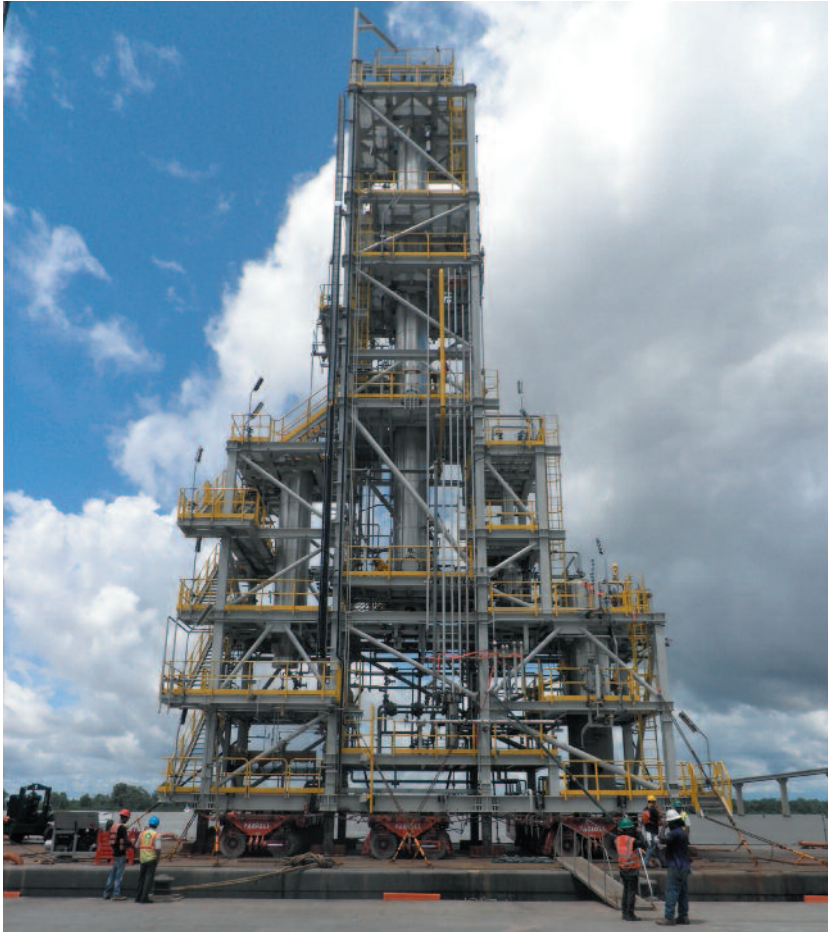
[Figure 9.8 – Load out project of a module]
