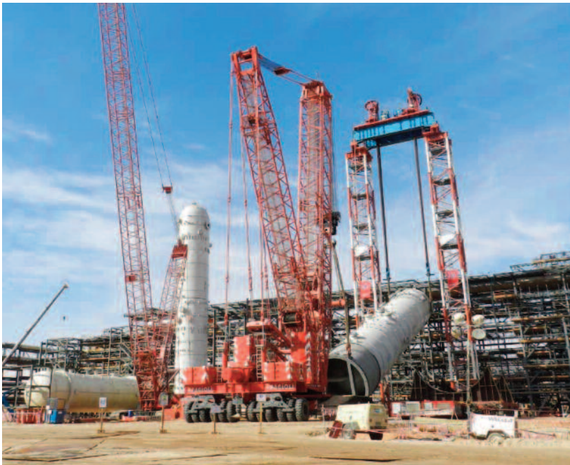
[Figure 8.6 – Reactor lifting Meg Project Singapore Foster Wheeler with Towers, Strand Jacks and Crane (Fagioli)]
