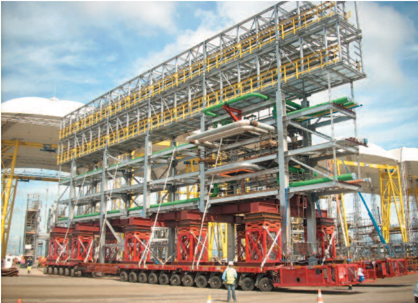
[Figure 11.3 – Module transport for Comperji refinery Brazil (Fagioli)]
