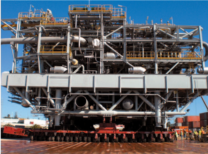
[Figure 10.4 – Load out project of a module]
