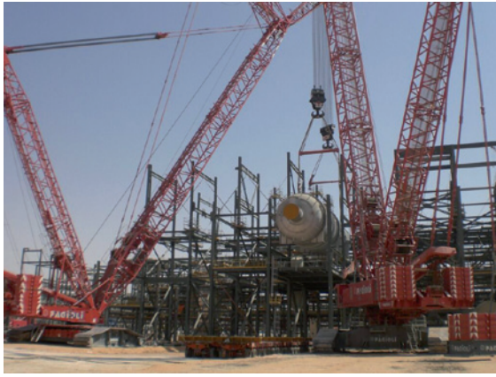
Fig. 2 - Reactor lifting Meg Project Singapore Foster Wheeler with towers, strand jacks and crane (Fagioli)
