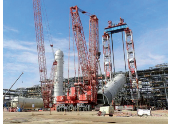
Fig. 2 - Reactor lifting Meg Project Singapore Foster Wheeler with towers, strand jacks and crane (Fagioli)
