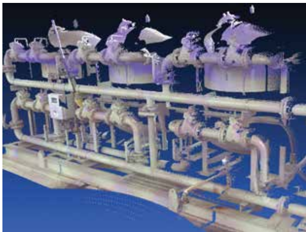
Fig. 2 - The point cloud is an accurate representation of the scanned plant
