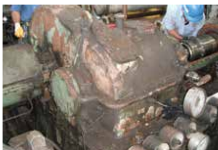
Images taken on site, before the overhaul
