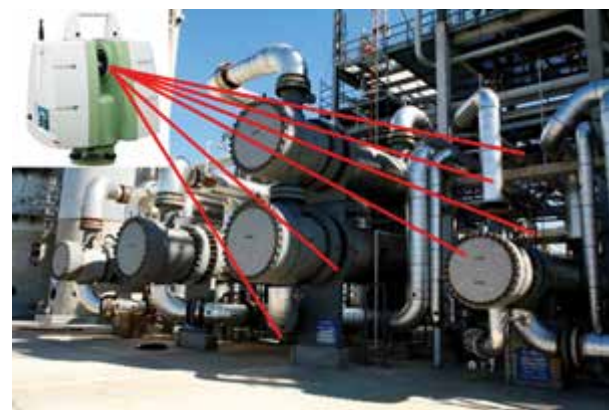
Fig. 1 - Within minutes the laser scanner takes millions of measurements
