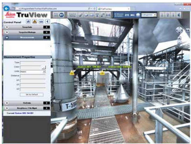
Fig. 3 - An example of a point cloud integrated with digital photographs.
