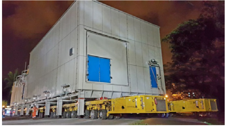
Substation module on SPMT
