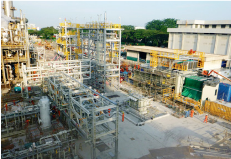
Cogen 2 site as it looked after the delivery of PAR/PAUs and before the arrival of HRSG
