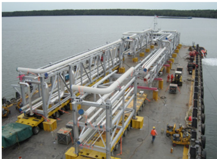
Legs-up PARs loaded on the barge
