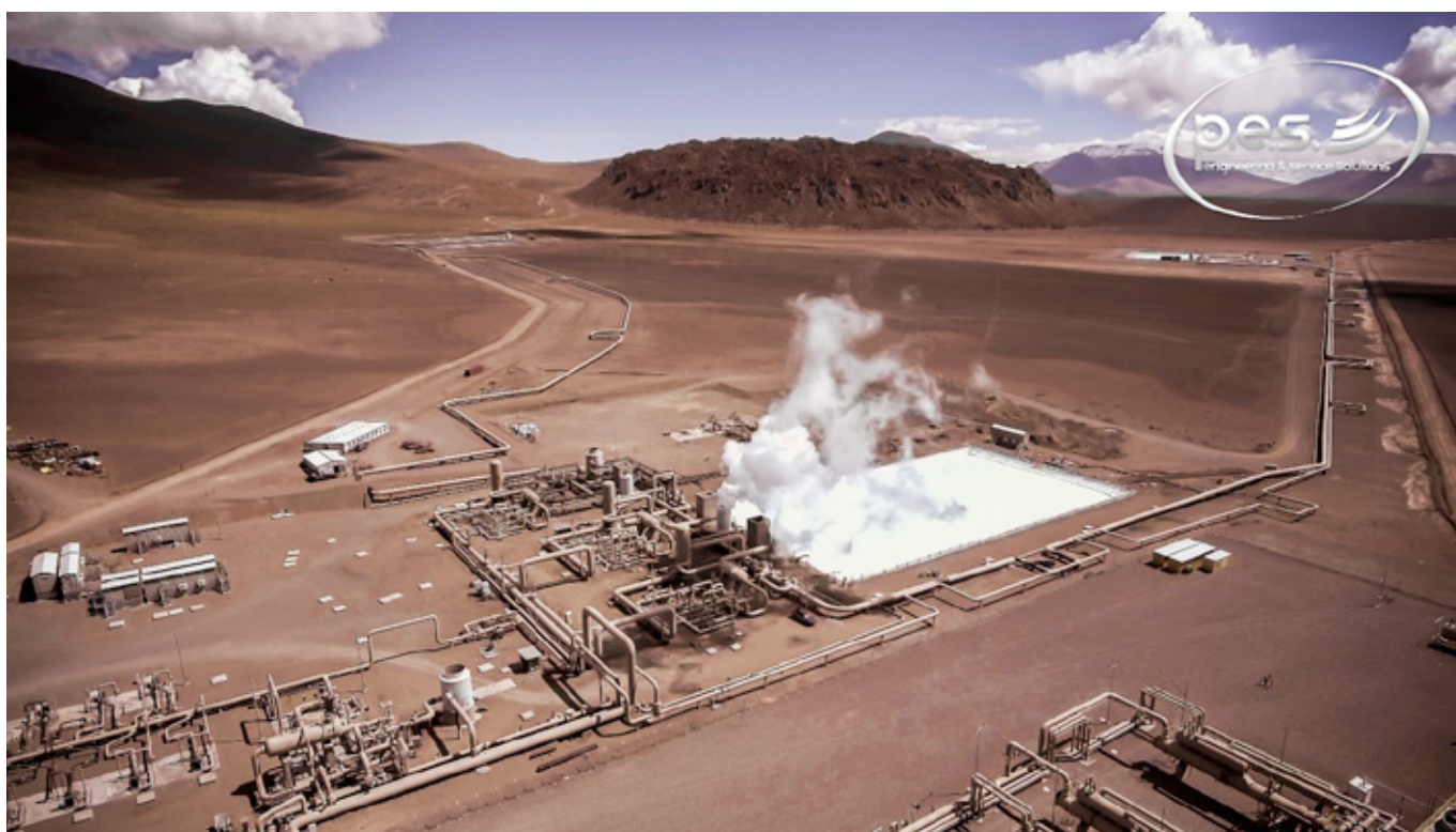
Figure 1: Reinjection Pump Station – Separation Station – Cp6 wellpad Overview
