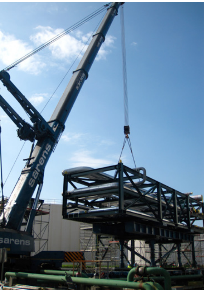
Lifting of interconnecting pipe-rack module
