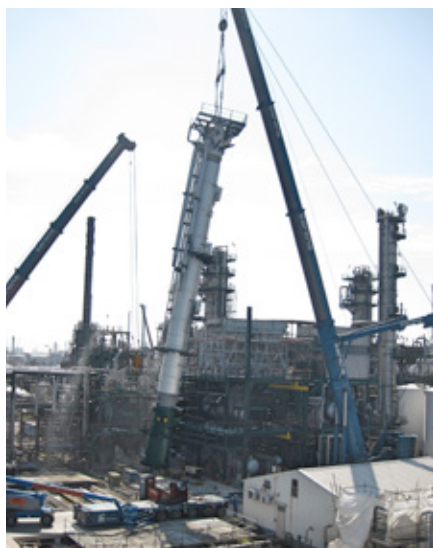
Lifting of SWS Column
