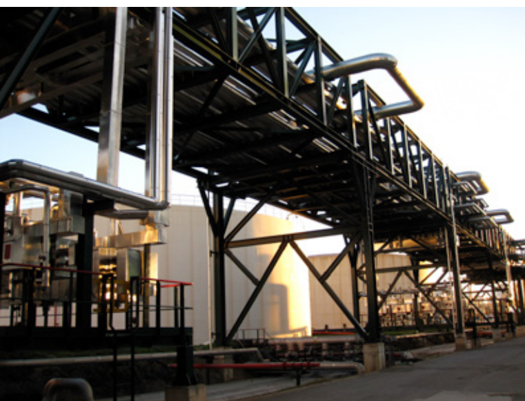
Interconnecting pipe-rack
