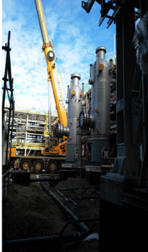
Figure 2 - Construction site of the gas storage plant "Corneghino Laudense Natural Gas"
