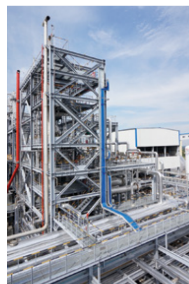
Side view of XLX Euromel® Melamine Plant, Xinjiang, China – World's largest single-train HP melamine plant, 60,000 ton/year
