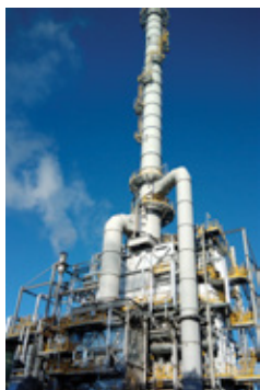
Steam Reforming Heater for Hydrogen Production Unit, designed and built in modularisation by Wood for KazMunaiGas Refinery at Atyrau, Kazakhstan Republic
