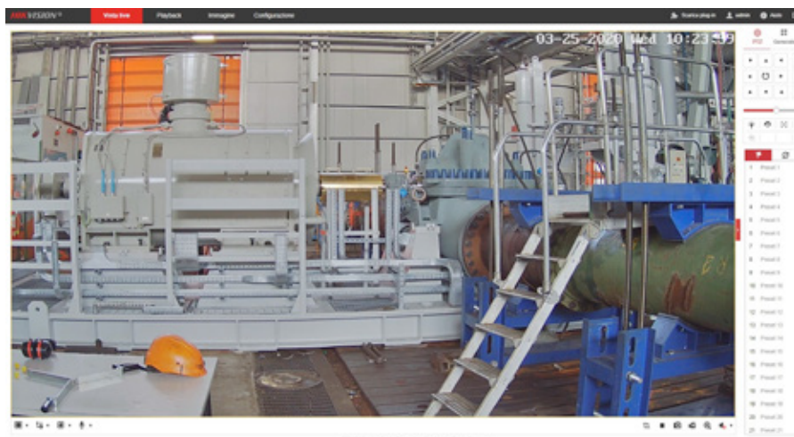
Web camera view of pump being tested
