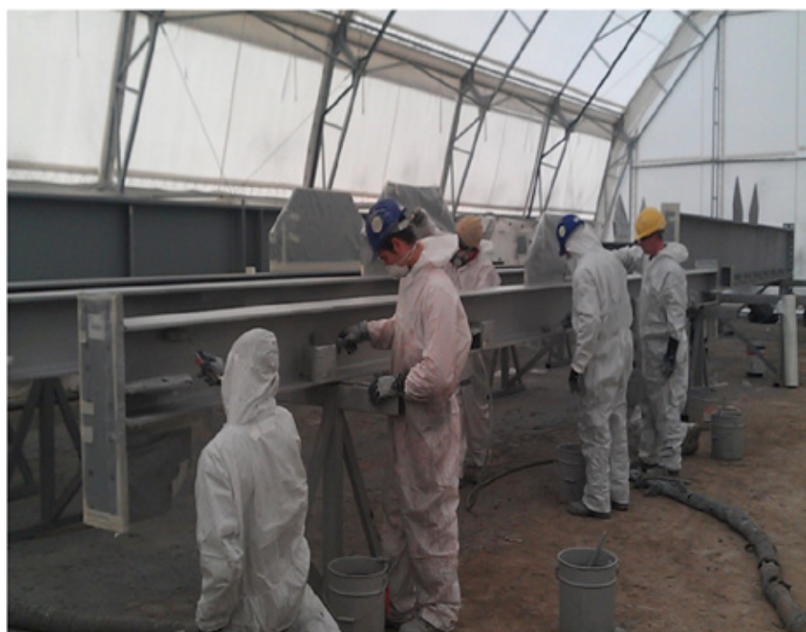
Figure 4 - Fireproofing treatment application at the Monsud S.p.A. plant in Avellino
